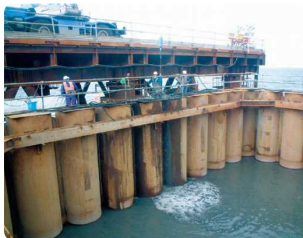
鋼管継手充填
